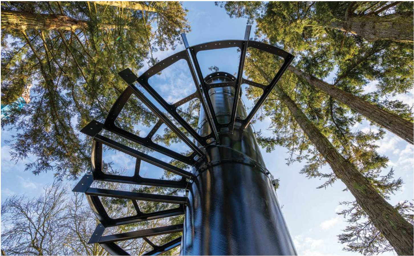
The Treehouse, which sits on one concrete footing, was designed and engineered to be lifted into existing mature trees.
