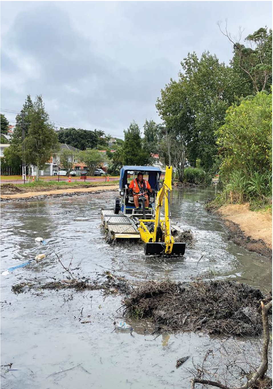
The project’s methodology centred on the adaptation of a suction dredging and dewatering technique from European wastewater dredging practices
