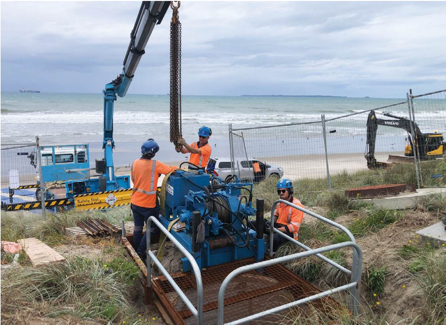
The pipe takes the treated water from the pump-station at the Te Maunga ponds to the sand dunes by way of a new 1.7km 1200mm pipeline.
