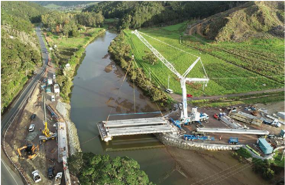
The delivery of the bridge beams to site and lifting onto the structure took about four weeks.
