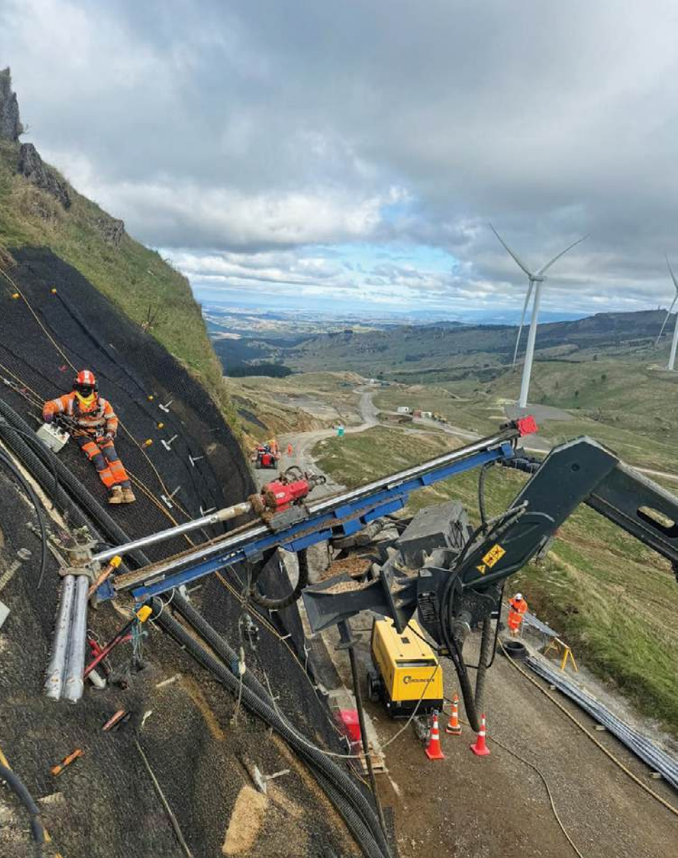
Groundfix staff work on cliff stabilisation at the Harapaki Wind Farm.
