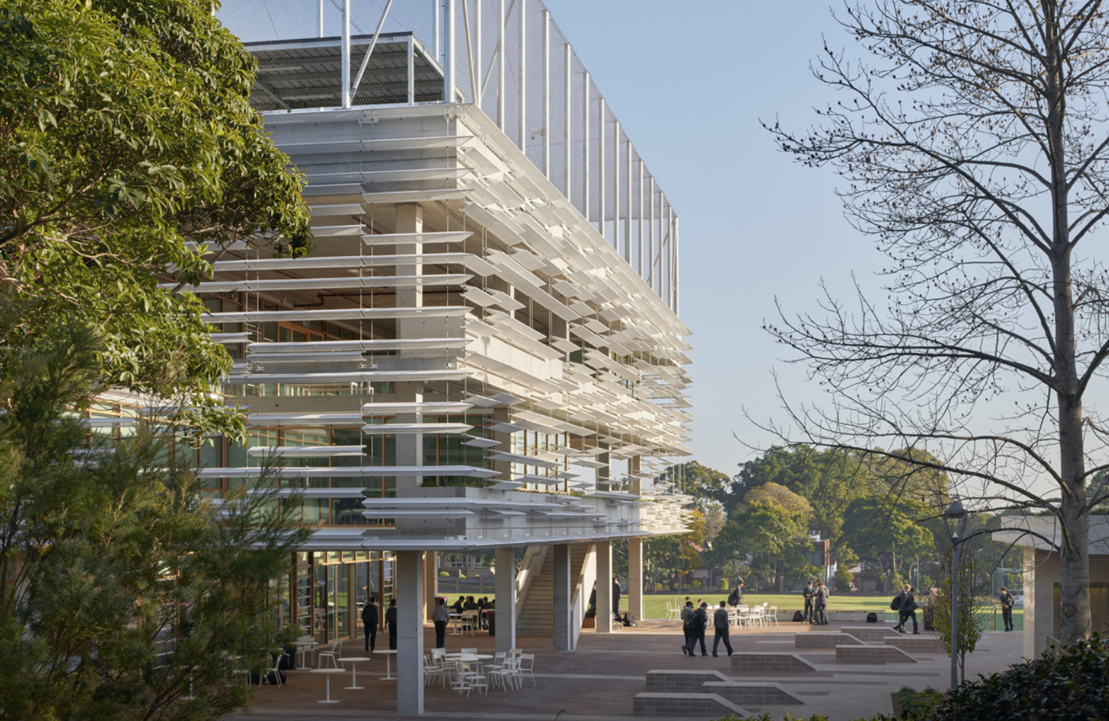
Image 4. Second skin Atmosphere facade of perforated aluminium panels supported by tensioned cables at St. Patrick's College in Strathfield.
