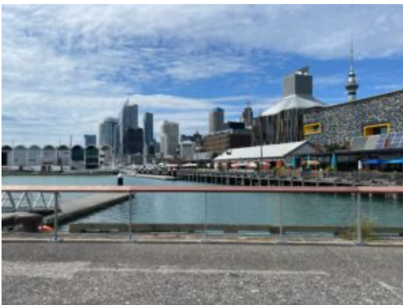
Looking East towards City Wharf Edge B02 C5 engineered with angled capping rail and ss mesh in-fill and baseplates
