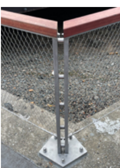
Custom Aperture Baseplate and Stanchion for change in direction
