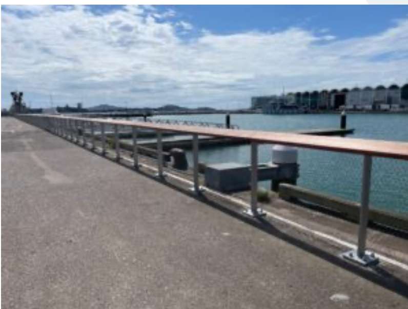
Wharf Edge B02 Design with angled capping rail and SS Mesh and Baseplates
